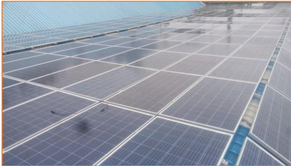
Solar plant installation in Bang Khun Thian factory.
